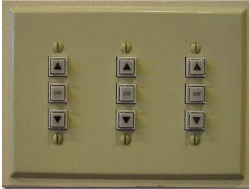
\*The wall controls for the screens have up and down arrows and a stop button. They are laid out as they are positioned in the rooms – the left button controls the left screen and so on.
