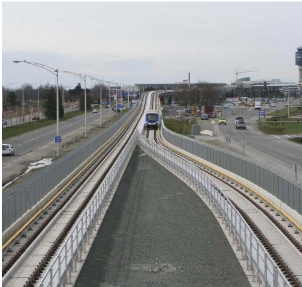
AT-GRADE SECTION TRACKWORK - YVR AIRPORT
