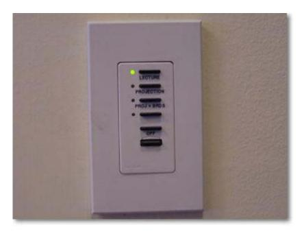
\*The Wall Controls have the following scene settings: Lecture, Projection, Projection & Boards and Off.
